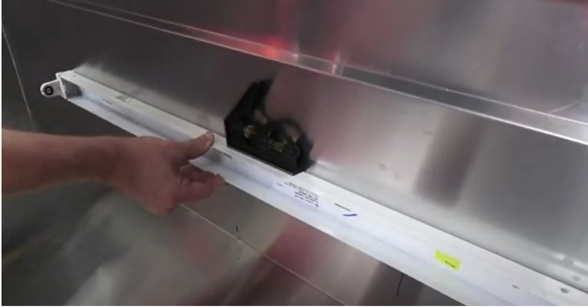
Figure B.14 Fluorescent light fixture leveled and in mount location
