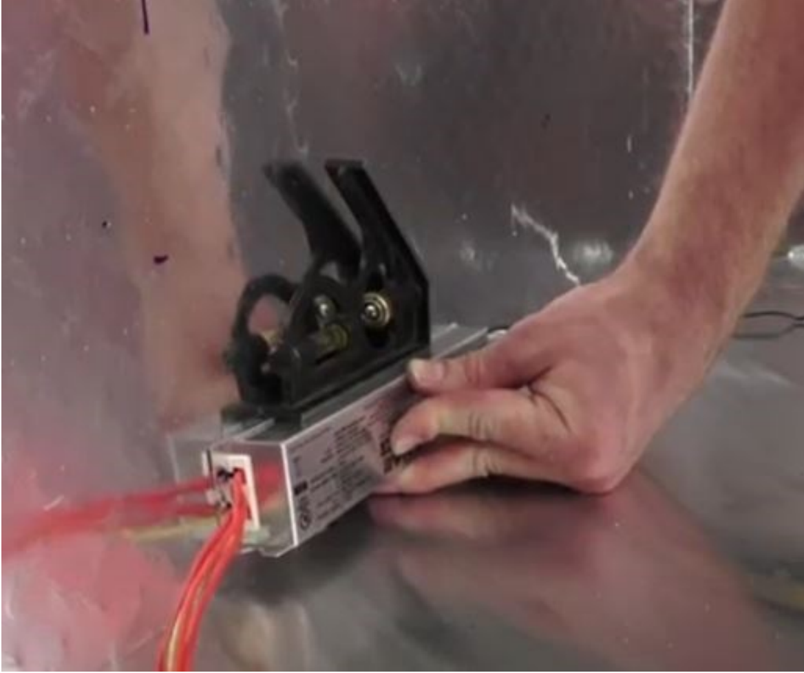
Figure B.12 Levelled workhorse ballast in mount location
