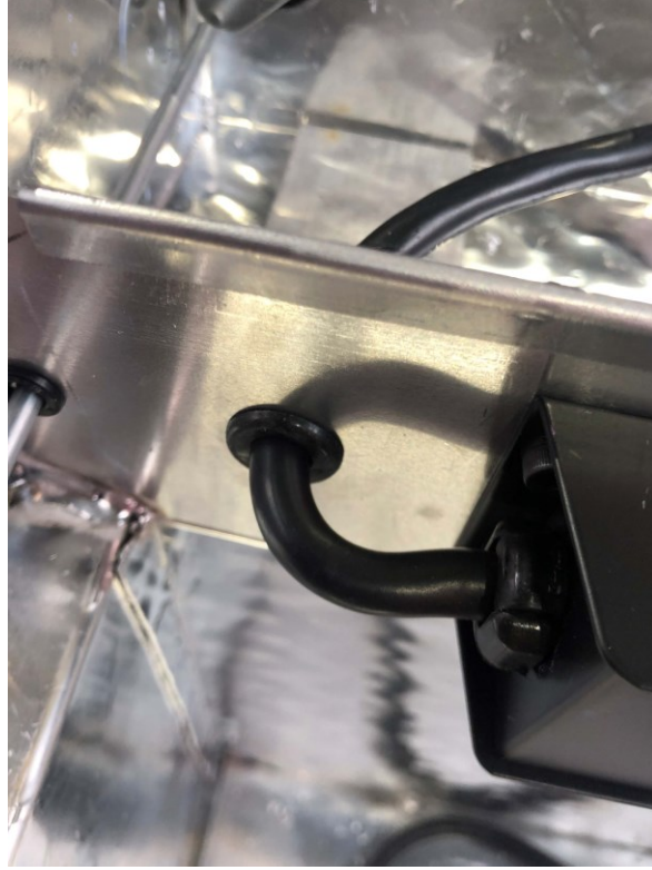
Figure B.8 The power cable of the power strip fed through the grommeted hole closest to the front of the toolbox
